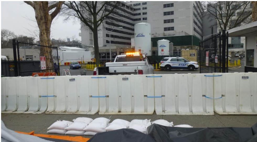
Figure 14 – Temporary floodwall deployed at a hospital site
