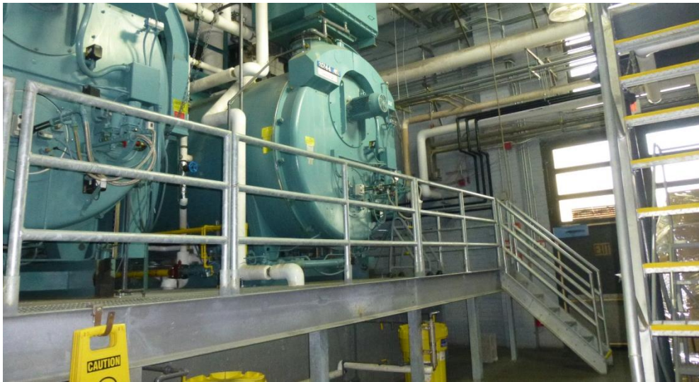
Figure 15 – Boiler system on elevated structure
