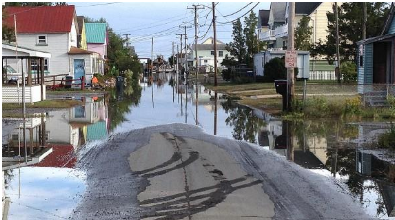
Figure 5 – Ponding due to runoff, Delaware (Bittle, 2015)
