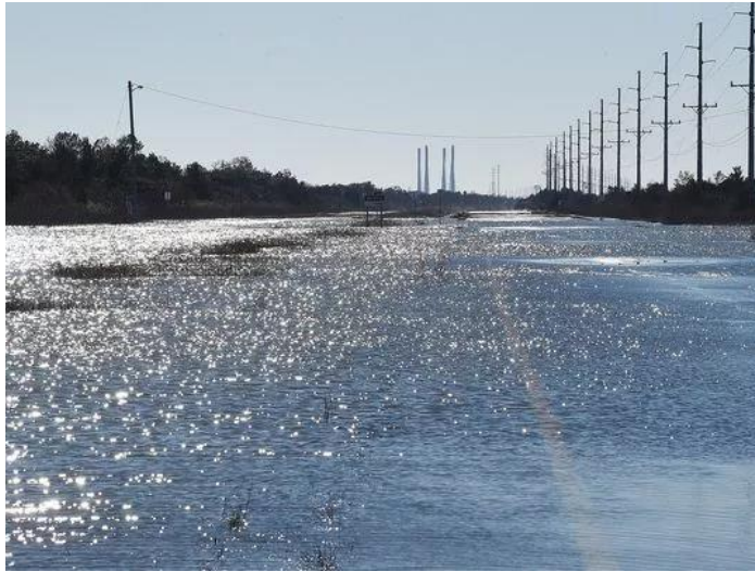
Figure 4 – Coastal flooding on Route 1, Delaware (Murray, 2017)
